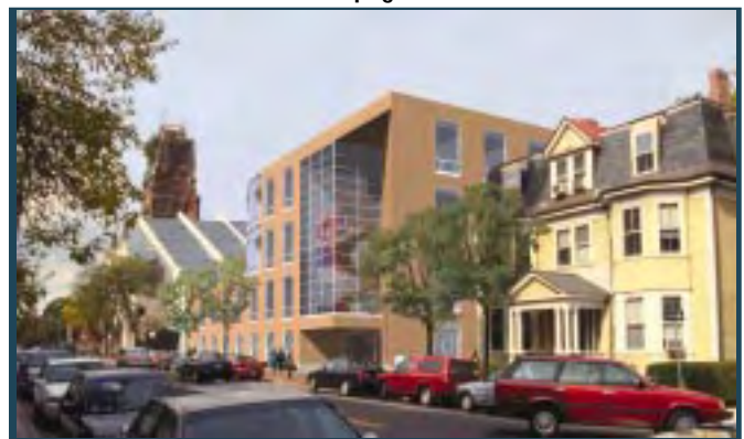
The Center for Government and International Studies (CGIS) will be the future home of the Weatherhead Center and will also house Harvard's Department of Government and centers for international study. The project began with a $2.1 million gift to the University from Sidney R. Knafel ('52), a member of the Center's Visiting Committee from 1991-2000.
